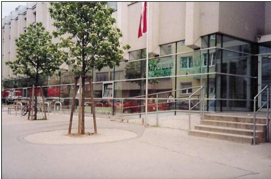
Fig. 7-1: Accessibility to school-buildings forms a major precondition for educational opportunities of children wD and their social and cultural integration (too steep ramp at Hauptschule in Vienna, 16 th district)
