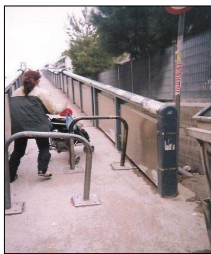
Fig. 15-11: Footbridge in Athens!!!
