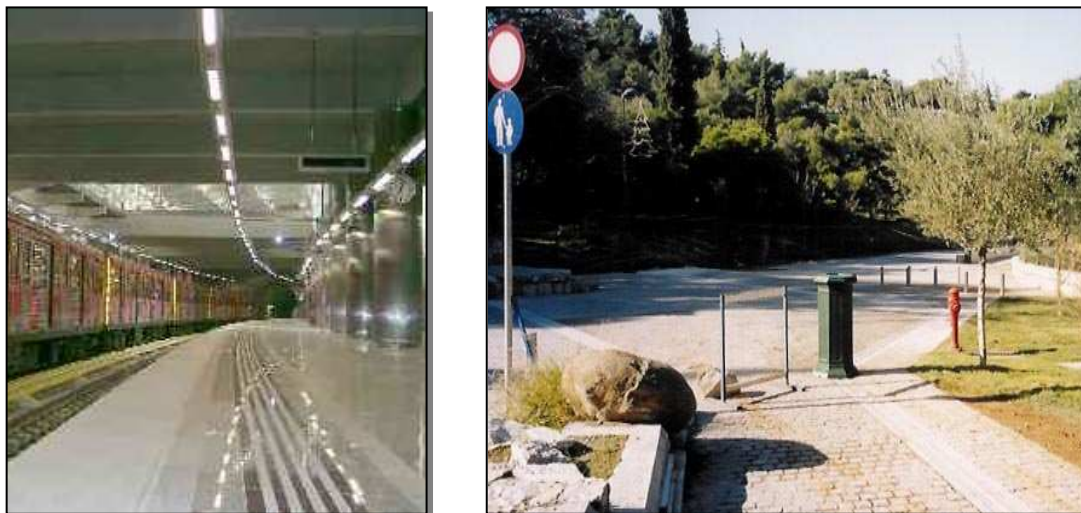
Fig. 11-66 and Fig. 11-67: Tactile orientation markings in a new Attiko Metro Station in Athens and on the Akropolis pedestrian zone on Apostolou Pavlou Street
