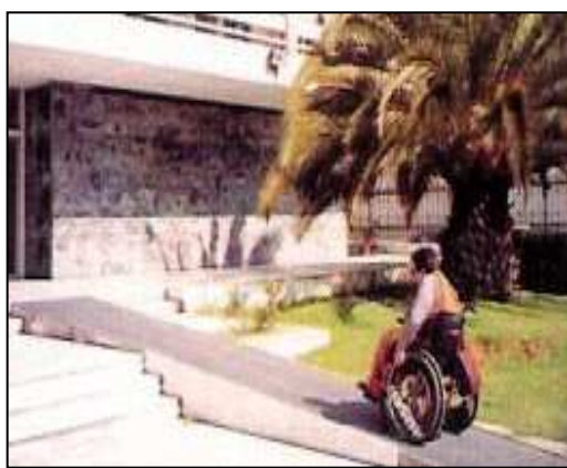
Fig. 15-8, Fig. 15-9 and Fig. 15-10: Some bad examples: ramps without railings or too steep inclinations
