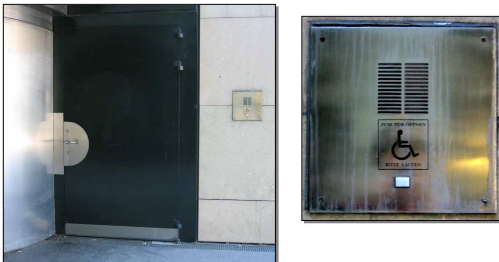
Fig. 12-8: 'Wheelchair users please ring for assistance!' – But the bell is obviously positioned out of reach for any wheelchair user!
