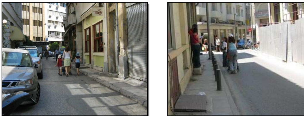
Fig. 15-27 and Fig. 15-28: Greek pavements are most prohibitive for the use of persons with any kind of chairs
