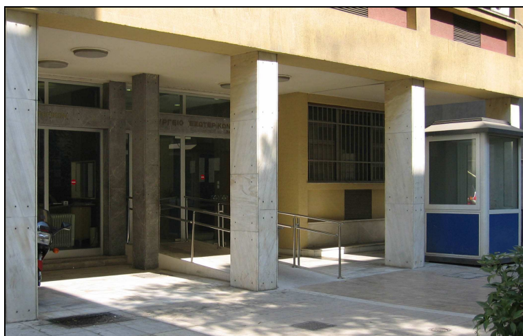
Fig. 15-2: Ramp with railing at the entrance of the Greek Ministry of Economy and Finance in Athens
