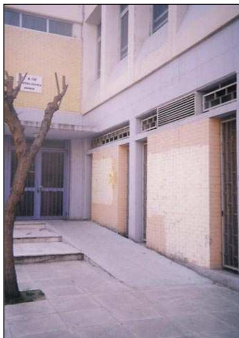
Fig. 7-4: All over Athens older public school-buildings have been adapted recently with ramps so as to become accessible
