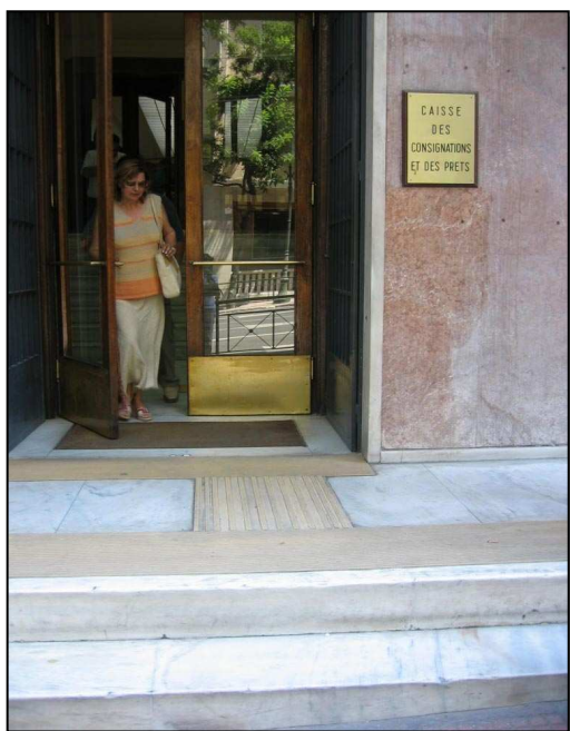
Fig. 15-3: Tactile orientation marking and curb cut at the entrance of the Cash of Consigns and Loans in Athens
