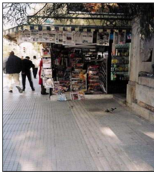
Fig. 8-2: Tactile orientation marking ending at an Athenian kiosk (city centre)!
