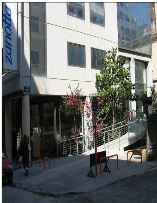
Fig. 15-7: Quite a rare sight in Athens: an private office building with a ramp – however, the ramp is much too steep to be driven up autonomously by a wheelchair user!
