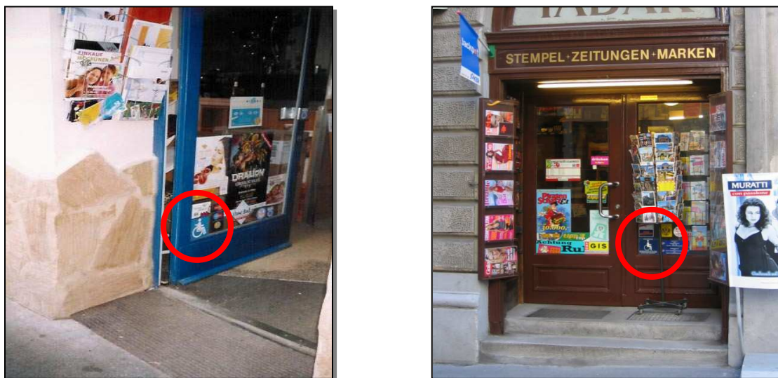
Fig. 14-4: Placing the International Sign of Accessibility on shop-doors does not always mean barrier-free access (ex. from Vienna)
