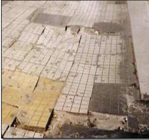
Fig. 14-16, Fig. 14-17 and Fig. 14-18: Badly constructed or yawning pavements are something 'ordinary' in Greece and can be found everywhere (ex. pavement with deep hole (up), loosened pavement covering (left) and sudden projection (right))
