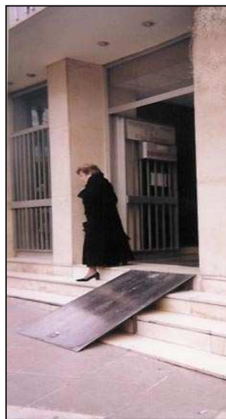
Fig. 16-11: The ramp at the Polykliniki Athinon
