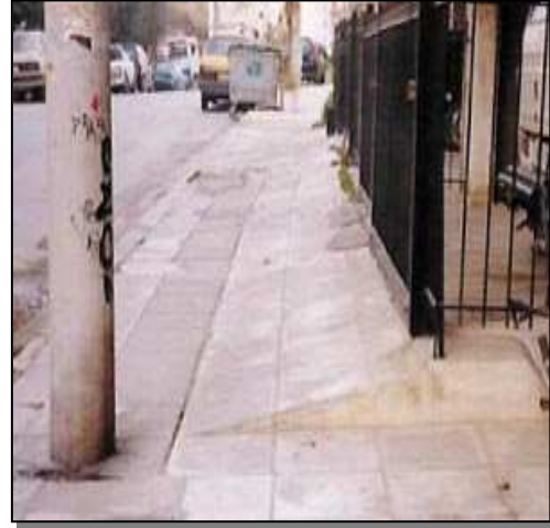
Fig. 14-16, Fig. 14-17 and Fig. 14-18: Badly constructed or yawning pavements are something 'ordinary' in Greece and can be found everywhere (ex. pavement with deep hole (up), loosened pavement covering (left) and sudden projection (right))
